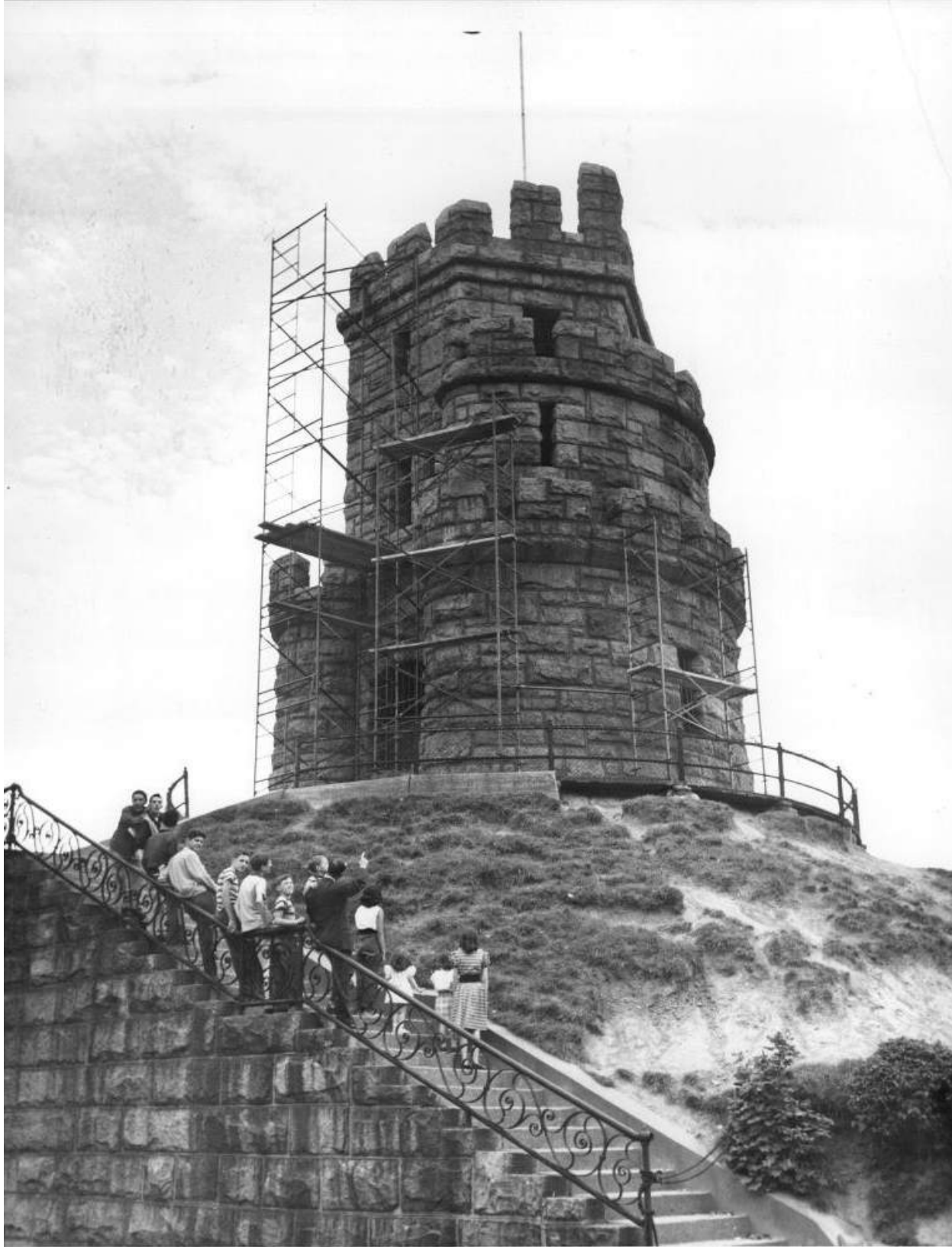
1954 erosion of slope supporting the tower
