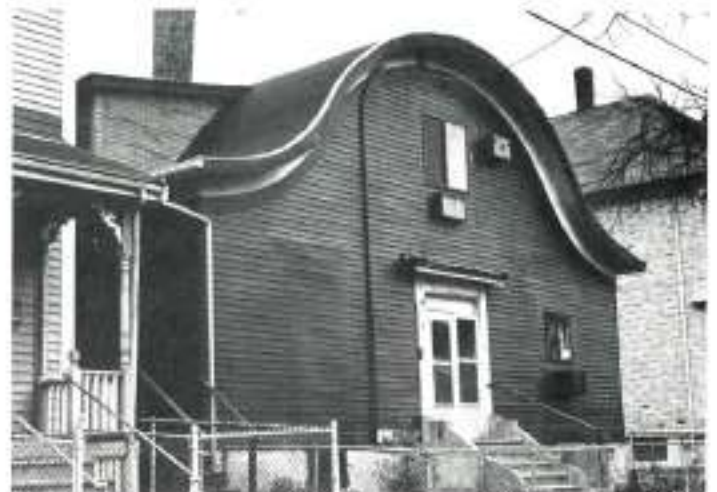
Philip Johnson House, 40 Trull Street, ca. 1868; moved ca. 1890. Originally situated at the corner of Medford and Central streets, this house stood at the top of a series of terraces. The unique roof survives, although other features have been altered. Philip Johnson was a florist.
