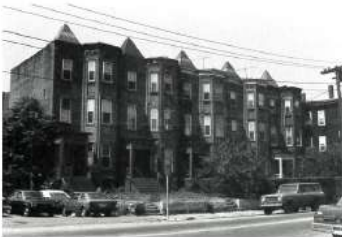
28-36 Beacon Street, ca. 1880. Built on land formerly owned by brickyard owner George Wyatt, this apartment row has five slate-covered pyramidal roofs, inset brick panels and decorative entrance porches.
