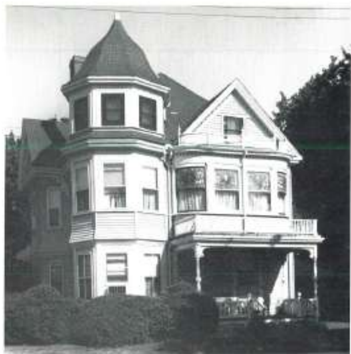
Charles H. Lockhardt House, 88 College Avenue, ca. 1890. Elm Street north of Davis Square was renamed College Avenue in the 1890s. A number of fine houses were built on College Avenue by Somerville businessmen, including Charles Lockhardt, an undertaker. This fine example of the Queen Anne Style, with curved panes of stained glass and a three-story corner tower, is also representative of houses built in the 90-lot William A. Russell subdivision which adjoins College Avenue.
