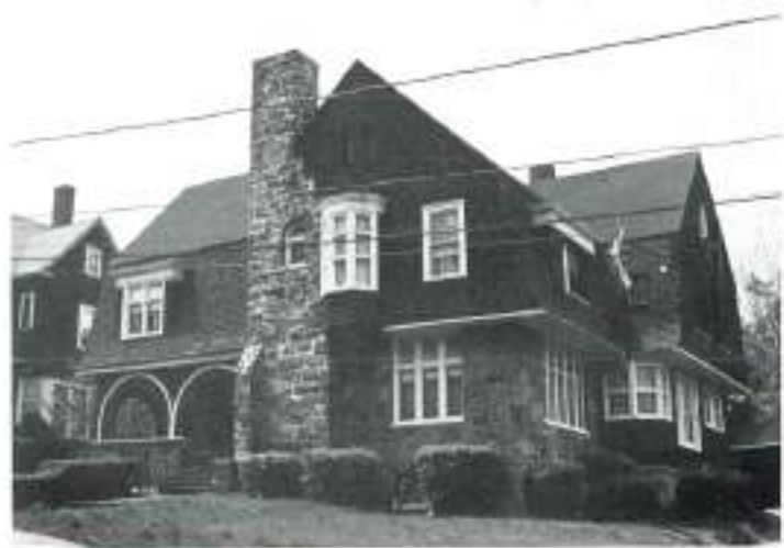
Eugene B. Carr House, 18 Benton Road, ca. 1910. Built for a partner in the M. W. Carr Company, Somerville manufacturers of jewelry and novelties, this Shingle Style house is in near-original condition, with a prominent fieldstone chimney mass and foundation and shingled wall surfaces.
