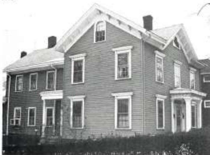
Frank Williams House, 37 Albion Street, ca. 1860. Albion Street (originally Forest Street) near Central Street has a row of Italianate houses built by businessmen in the 1850s. Frank Williams was a Boston kitchen furnishings dealer. 37 Albion retains its distinctive trefoil windows in the front gable, and an ornate porch and window enframement.
