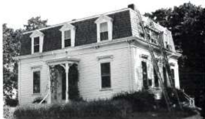
30 Day Street, ca. 1870. Patterned slates are an intact feature of this mansard-roofed house near Davis Square.
