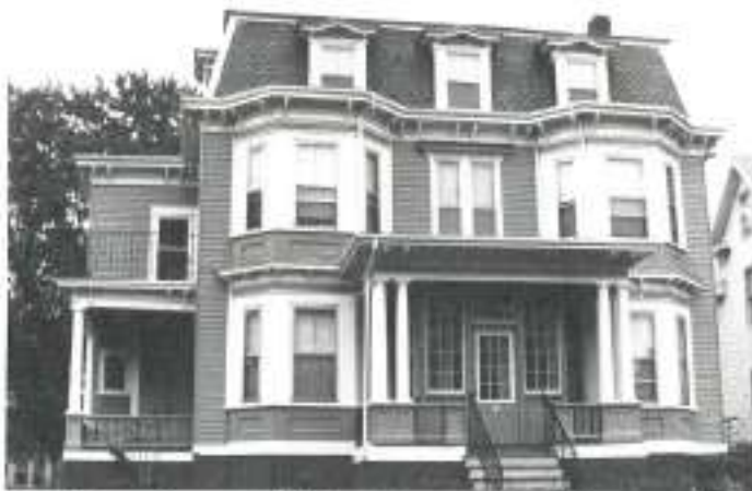
John E. Ayer House, 141 Walnut Street, ca. 1870. This mansard-roofed house was built by Charlestown lumber dealer John E. Ayer. Ayer also sold land in Somerville.
