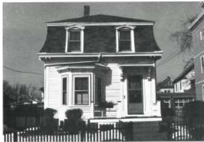
53 Moore Street, ca. 1870. This dwelling is among a collection of early mansard-roofed houses on Clarendon Hill. It was first the home of railroad workers Robert J. and George C. Melville, and later Granville M. Edwards, a blacksmith.
