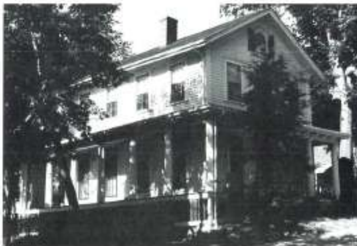
Amos Keyes House, 12 Adams Street, ca. 1845. This house was built by produce dealer Keyes on Central Street, and moved to Adams Street when Keyes constructed a new house about 1870. The second Keyes residence, a once high-styled mansard house, is situated at 152 Central Street.
