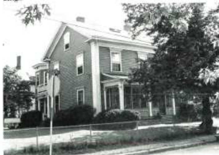
24 Chester Street, ca. 1858. This early Davis Square area house retains wide, grooved cornerboards which are part of the original Italianate design.
