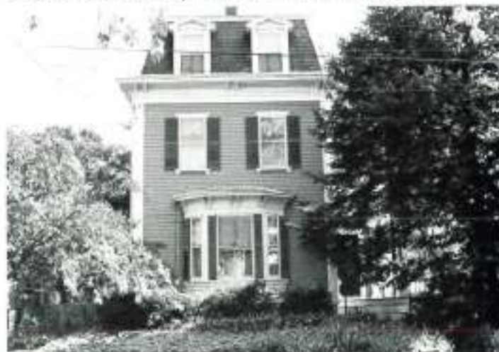
26 Chester Street, ca. 1878. A slate-covered mansard roof is an original feature of the Second Empire treatment of this three-story house.
