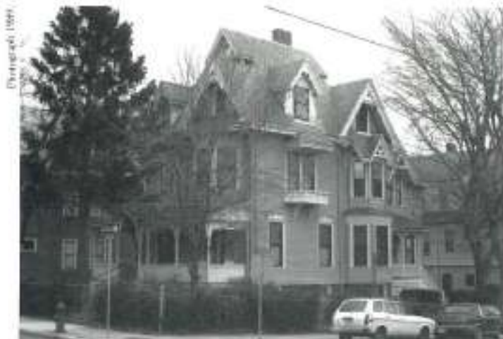
Otis-Wyman House, 67 Thurston Street, ca. 1883. Although the original clapboard siding has been covered over, the Otis-Wyman House is one of the city's exceptional late nineteenth-century residences. Most of the original decorative trim, including a picturesque roofline with numerous hooded dormers and cusped bargeboards, is intact. Built in the Strickney subdivision at a time when the area was rapidly becoming the home of Boston and Somerville businessmen, this was the residence of William R. Otis, a cabinetmaker, and later Charles B. Wyman, a restaurant owner.
