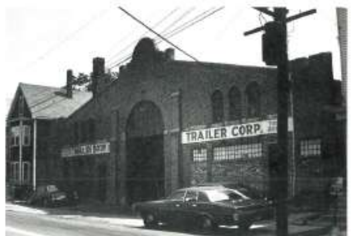
Automobile Repair Garage, 94 Prospect Street, 1917.
