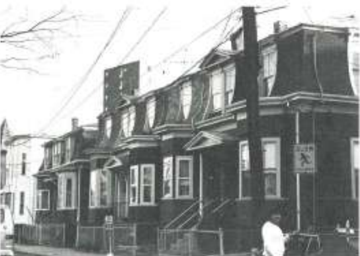
26-32 Houghton Street, ca. 1860. Between 1854 and 1859, Amory Houghton, proprietor of the Union Glass Works, platted lots in Ward II for the construction of glassworker's and artisans houses. These mansard rows were among the first buildings in the subdivision.
