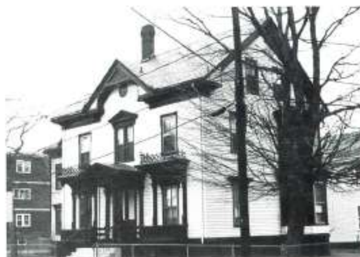
Nathan Tufts-Charles Williams, Jr. House, 1 Arlington St., ca. 1858. 1 Arlington Street is an excellent example of an Italianate house with later Eastlake Style trim. 1 Arlington was also the terminus of the world's first outdoor experimental telephone line. Charles Williams, Jr. bought the house from Nathan Tufts in 1876. Williams was a protege of Alexander Graham Bell, and Bell and Watson's first telephone was developed in 1875 at Williams' electrical shop at 109 Court Street, Boston.
