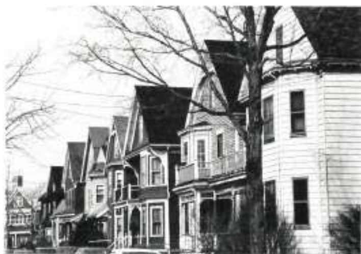
Campbell Park, ca. 1890–1900. Campbell Park, in the subdivision known as Campbell Park, is representative of building types and Queen Anne architectural styles found in many late nineteenth century Somerville subdivisions. Campbell Park was considered a suburban neighborhood by its many early residents who worked in Boston and used the trains and streetcars which stopped at Davis Square stations.
