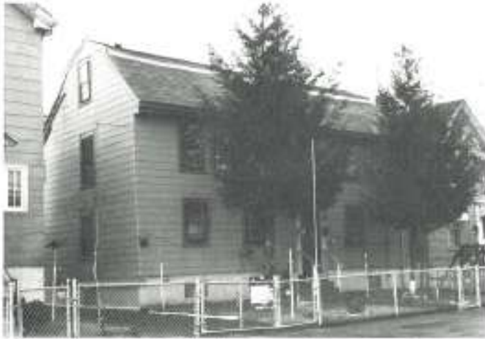
6 Kent Court, ca. 1750. This five-story, gambrel-roofed Colonial house was moved to its current location from Somerville Avenue. Nearby, Kent Street was an early connector between Beacon Street (1813) and Milk Row. After the Civil War, Kent Court was squeezed between the Reitenbach Brothers Mink Tannery, the Middlesex Bleachery, and the tracks of the Fitchburg Railroad.
