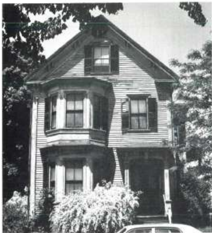
48 Vinal Avenue, ca. 1874. This gable-roofed, Italianate Style house has paired brackets at the eaves, a two-story projecting bay, and rope-beaded moldings at the corner boards. The lot was subdivided by Robert Vinal from Ira Hill's plan of 1870. Builders Silas and Emma Parker sold it to James and Sophia Burnett. Burnett was a machine blacksmith in Boston.
