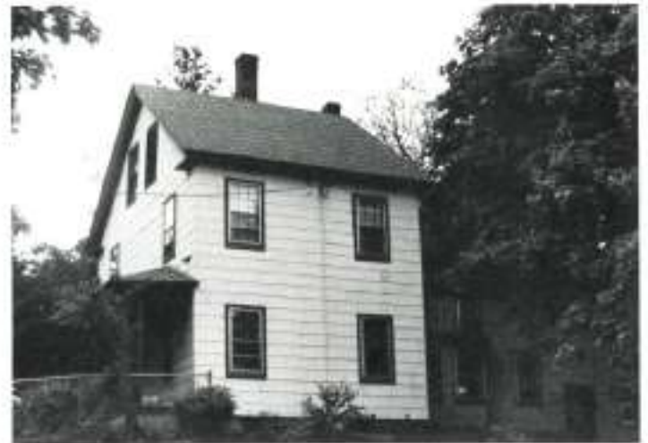
Simon Holden House, 97 Curtis Street, 1863. Another survivor of the early Curtis Street rangeway, this Greek Revival house was built by a market gardener. Another Greek Revival farmhouse is located at 21 College Hill Road, where it was moved from its original North Street site.
