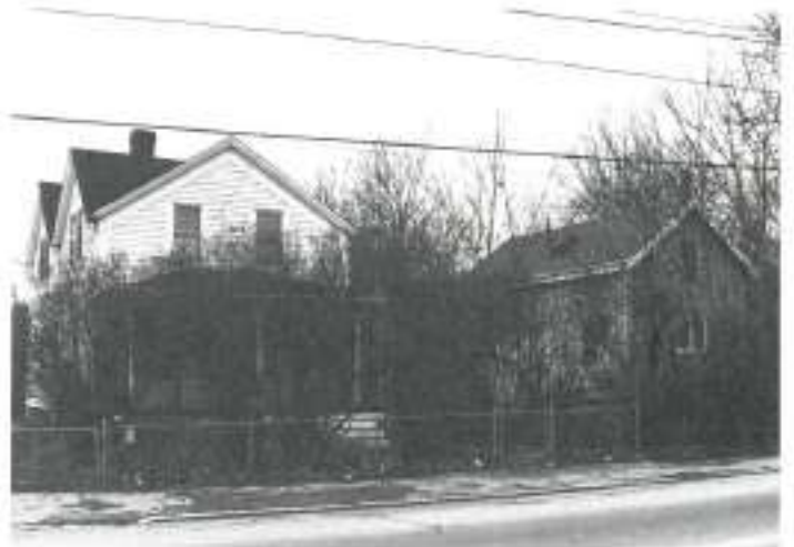
336, 338 Beacon Street, ca. 1840. Beacon Street was built in 1813. This pair of houses are among the earliest remaining buildings. 336 is of Greek Revival derivation, with a sidelit entry; 338 has a cusped bargeboard and steeply pitched gables characteristic of the mid-century Gothic Revival style.
