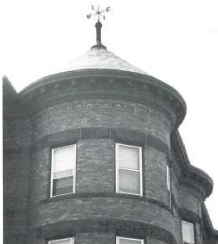
The Highland, 66 Highland, 1892. Samuel Dudley Kelley, architect. Boston architect Kelley was a noted designer of apartment buildings. His 1892 design for the Highland was advertised throughout the Boston area. The brownstone-trimmed brick building was finished with marble entrances, tile floors, and oak trim and offered excellent views from its Central Hill site.
