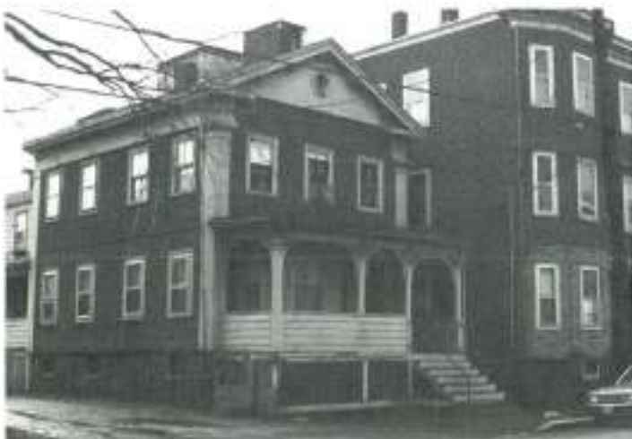
384 Washington Street, ca. 1855. Washington Street near the Cambridge line (and Kirkland Street) was once a corridor of fine homes on spacious lots. This house, owned by jeweler Charles Schuebeler in 1869, has an array of intact original details which surround the twentieth century asphalt siding. Of particular significance is the central oculus surrounded by a carved wooden garland.
