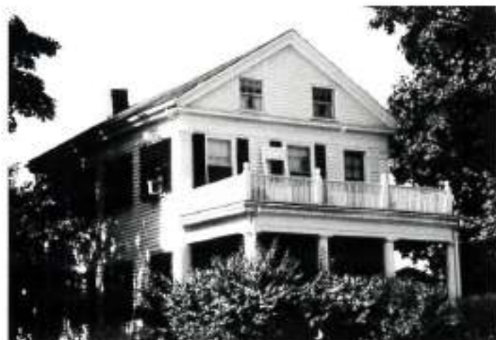
Adams-Locke House, 178 Central Street, ca. 1840. This house, an excellent example of the Greek Revival style, was built for Charles Adams, a farmer, Quincy Market merchant, and state legislator. A later resident, Woodbury Locke, was a Boston leather dealer.
