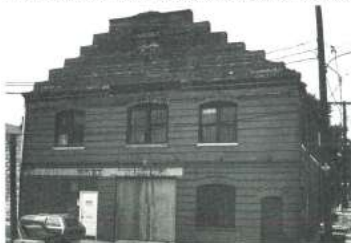
Walker Garage, 88 Winslow Avenue, 1911. Andrew Walker constructed this brick and terra cotta automobile repair garage in 1911. The two-story garage has a high stepped parapet with 17 courses of ornamental terra cotta cornice tile. Today, the garage serves as a sculptor's studio.
