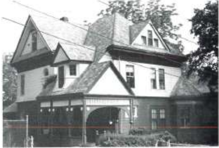
49 Spring Street, ca. 1893. George E. Loring, architect. One of five Queen Anne houses built on a subdivided estate by Christopher Rymes, a partner in the machine manufacturing firm of Cook, Rymes, and Company. Original details of this example are intact, including an elaborate porch with bulbous, turned posts.
