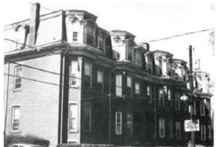
192–200 Central Street, ca. 1880. Like its neighbor at 55 Adams Street, this five-unit apartment row was built by real estate dealer and Winter Hill resident Curler Downer.
