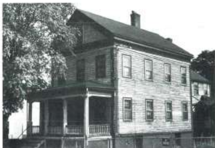
H. M. Hutchins House, 16 Mt. Vernon, ca. 1850. Harrison M. Hutchins was a "whitener" (bleachery employee) who worked for a Boston firm, according to the 1869 Directory of Somerville, Arlington and Belmont . The Hutchins House is an excellent example of the three-bay Greek Revival house found in East Somerville. A Doric-columned porch, 6 over 6 sash, and pedimented gable are features of the original design.
