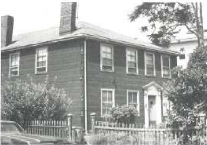
Cooper-Davenport Tavern, 81 Eustis Street, 1808. This Federal period building was originally a part of the Cooper-Davenport tavern on Beech Street in Cambridge. This portion of the tavern (an 1808 addition to the original 1757 tavern) was moved to Somerville in 1885. The pedimented entrance with slender pilasters is of note.
