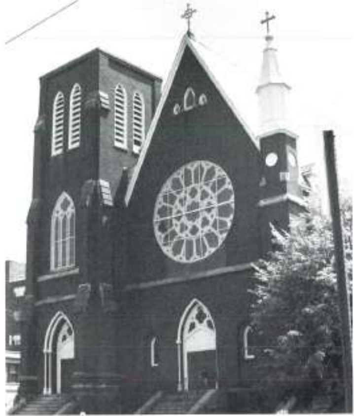
St. Joseph's Church, Washington Street and Union Square, 1874. James Murphy, architect. The city's first Catholic Church retains its original tower and spire. A high-styled Second Empire Style house (ca. 1875), now a rectory, and a ca. 1890 three-story school (ca. 1890) complete the church complex.
