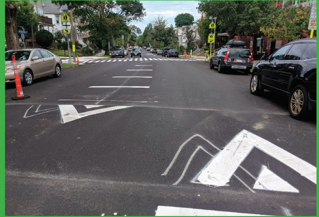
Speed humps on Powder House Boulevard
