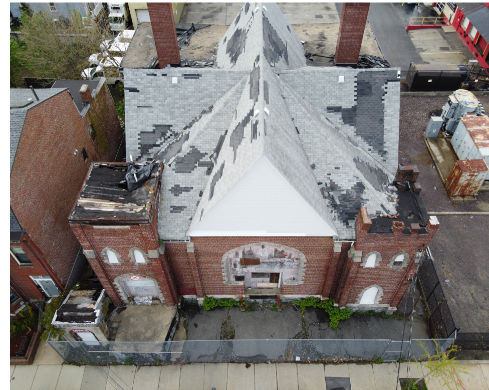
24 CROSS STREET EAST
