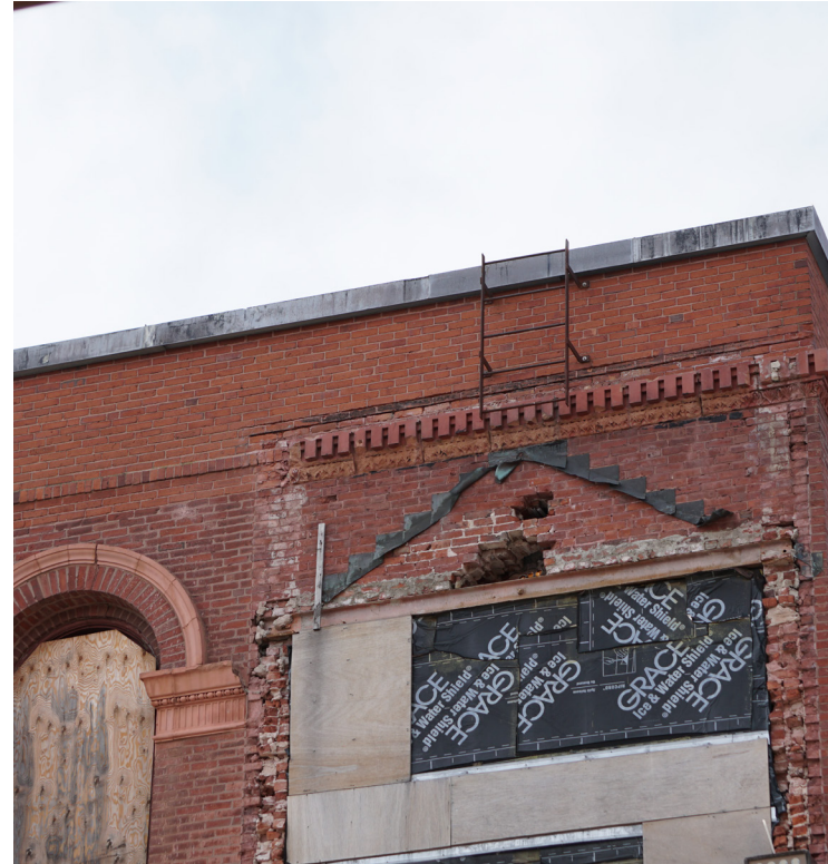
1895 BUILDING Openings exposed to the elements
